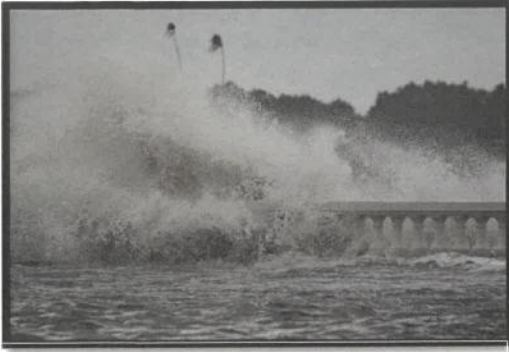
June 2012 Tropical Storm Debby/Bayshore Boulevard
