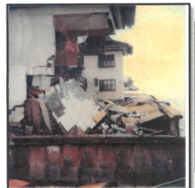
Hurricane Elena Damage 1985
