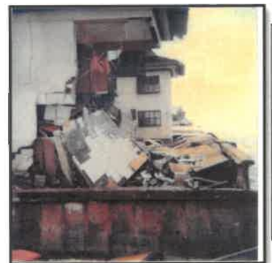
Hurricane Elena Damage 1985
