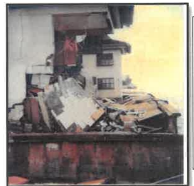
Hurricane Elena Damage 1985
