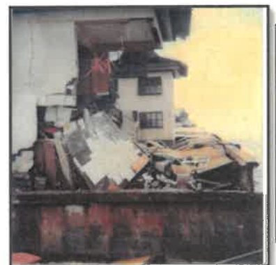
Hurricane Elena Damage 1985
