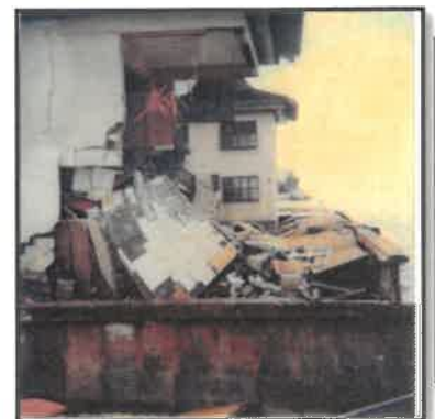
Hurricane Elena Damage 1985
