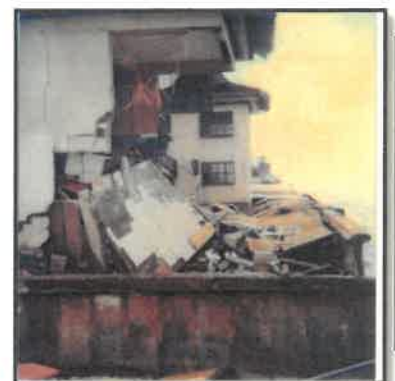
Hurricane Elena Damage 1985
