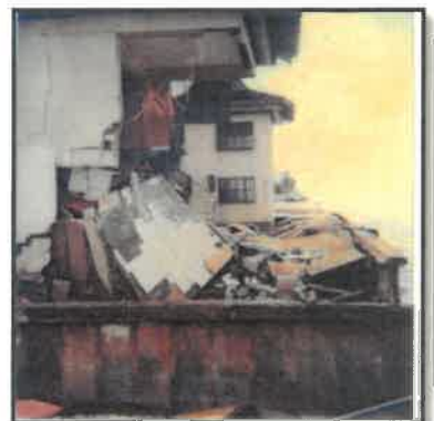
Hurricane Elena Damage 1985
