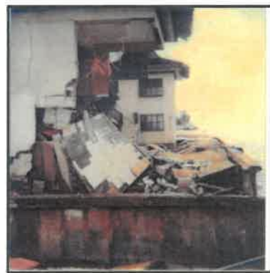
Hurricane Elena Damage 1985
