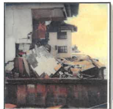
Hurricane Elena Damage 1985
