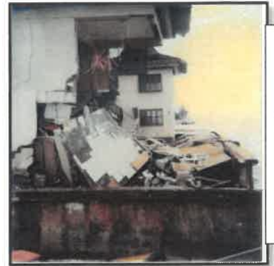
Hurricane Elena Damage 1985
