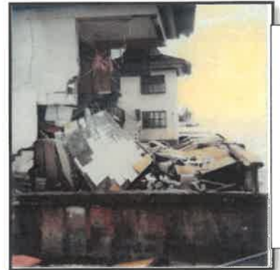
Hurricane Elena Damage 1985
